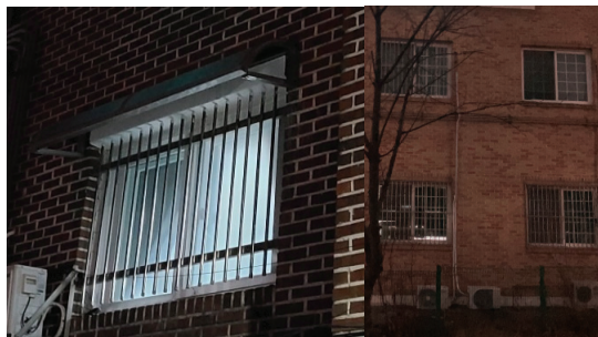
Fig. 15. Crime prevention bars on lower floors
