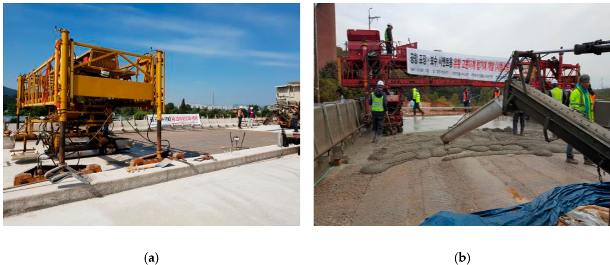
Figure 19. Further field study on the application of HMS concrete pavement. (a) Tanchon bridge, Republic of Korea. (b) Mandeok IC, Republic of Korea.
