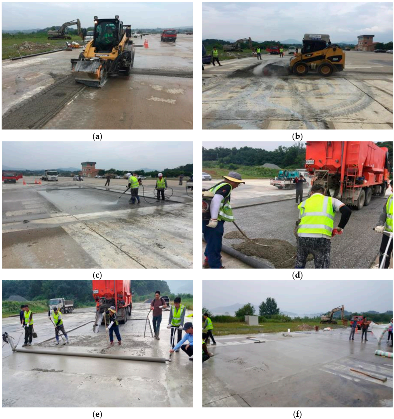
Figure 5. (a) Removal of old concrete pavement, (b) cleaning, (c) surface treatment, (d) casting of HMS concrete pavement, (e) finishing, and (f) curing.
