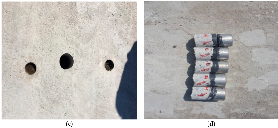
Figure 18. Results of 3 months of field monitoring. (a) Visual inspection, (b) sample cores, (c) core drilling, and (d) pavement inside testing.
